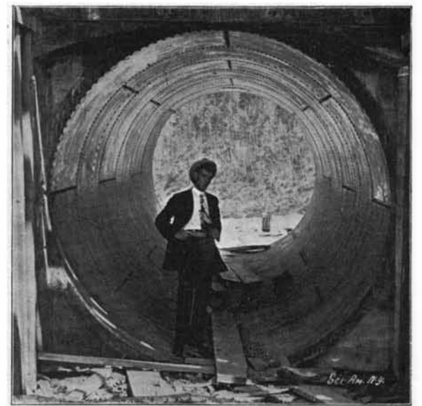
INSIDE PENSTOCK—9 FEET IN DIAMETER.
