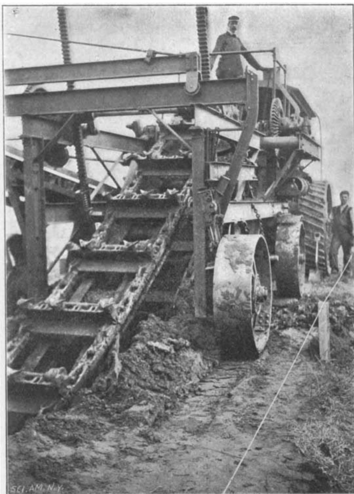
A VIEW SHOWING ENDLESS CHAIN WITH BUCKETS.
