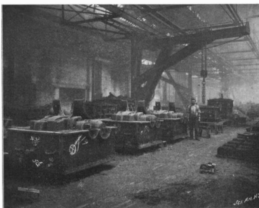
The Foundry, Showing Flasks for Compound Cylinders.
