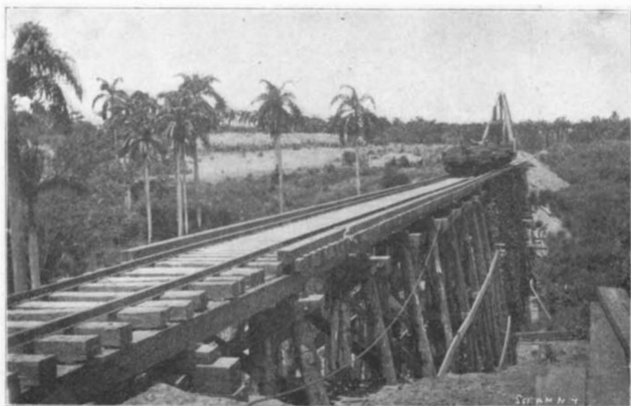
Pile Trestle Bridge on the Eastern Division.
