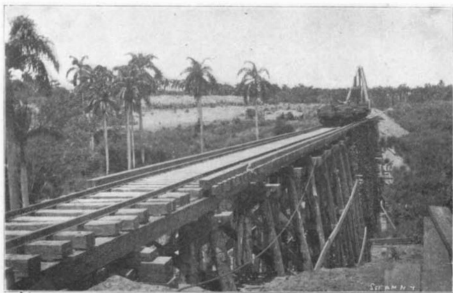
Pile Trestle Bridge on the Eastern Division.
