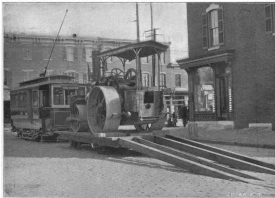
STREET ROLLER READY FOR TRANSPORTATION.
