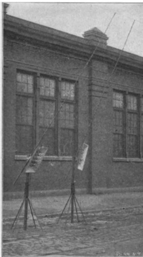
PORTABLE LIGHTS FOR CONSTRUCTION AND REPAIR WORK.
