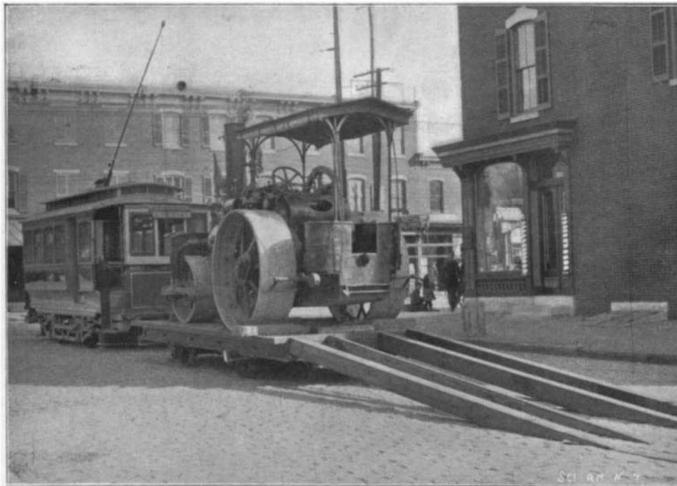
STREET ROLLER READY FOR TRANSPORTATION.
