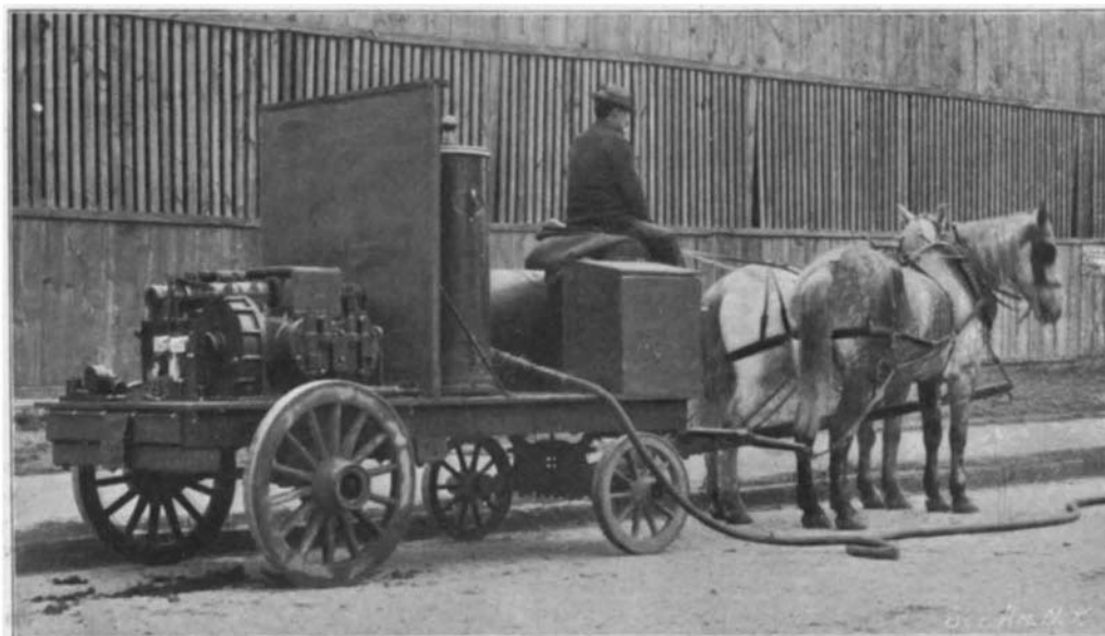
PORTABLE WELDING MACHINE, WITH ASBESTOS SCREEN FOR PROTECTING OVERHEAD WORK.
