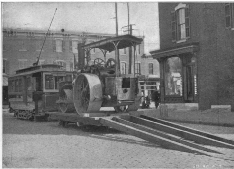
STREET ROLLER READY FOR TRANSPORTATION.
