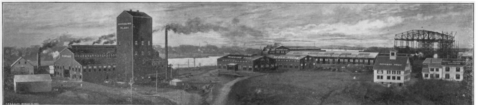
A GENERAL VIEW OF THE FORE RIVER WORKS.
