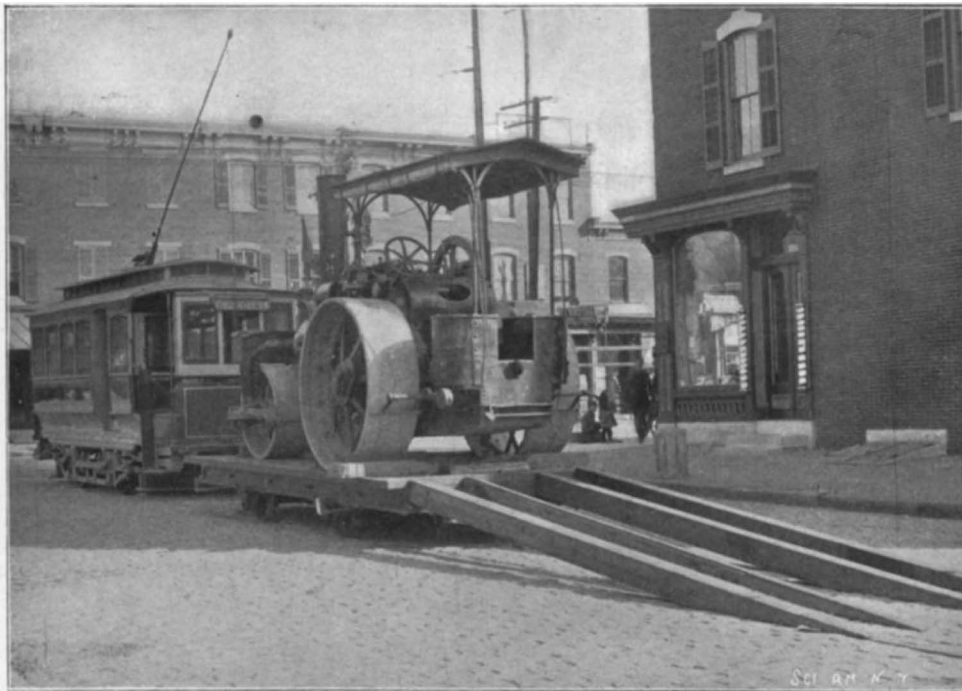
STREET ROLLER READY FOR TRANSPORTATION.
