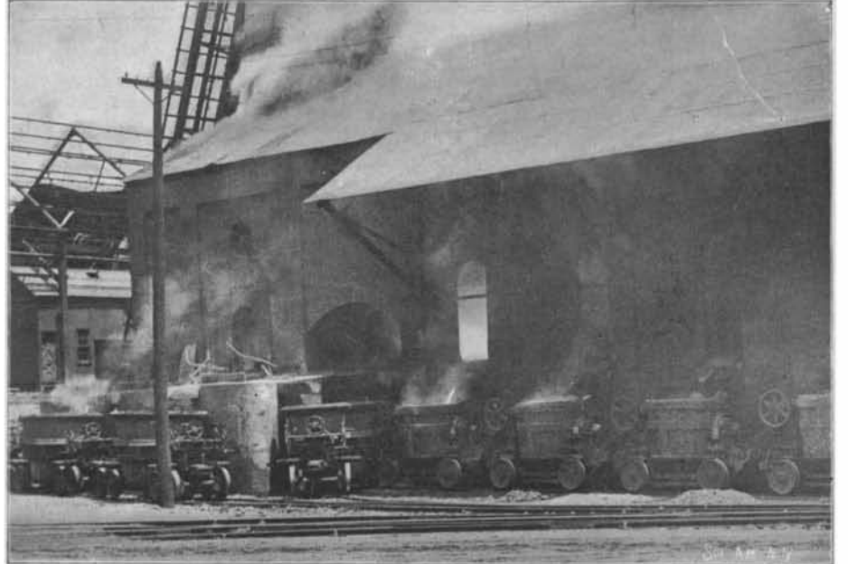
Tapping Contents of Blast Furnace Into Ladles.
