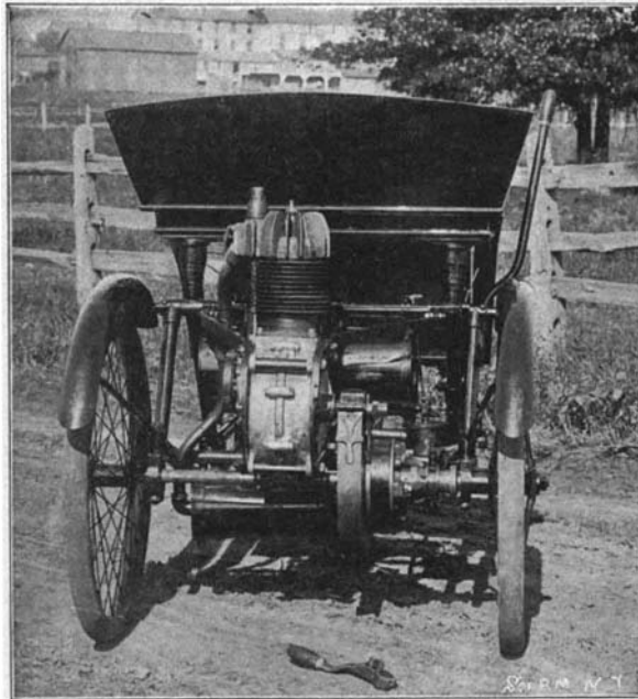
REAR VIEW, SHOWING MOTOR OF THE TURNER THREE-WHEELER.
