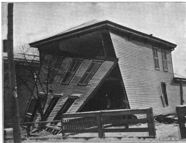
A HOUSE AT FORT WAYNE, IND., PARTIALLY DESTROYED BY AN ACETYLENE GAS EXPLOSION.
