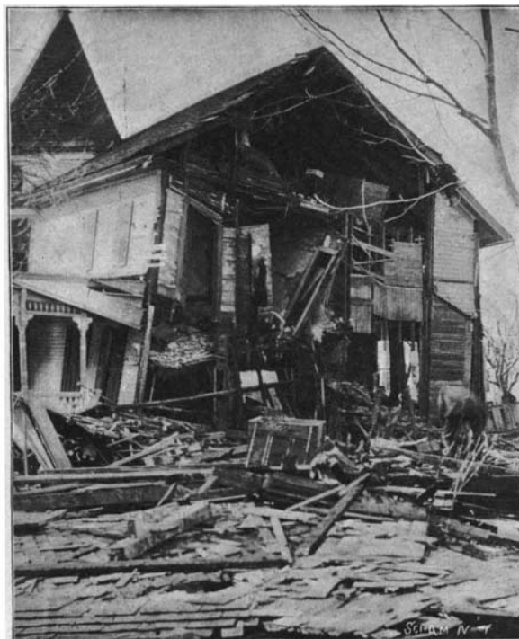
A RESIDENCE IN WEST BROOKFIELD, MASS., ALMOST DEMOLISHED BY A GAS EXPLOSION.
