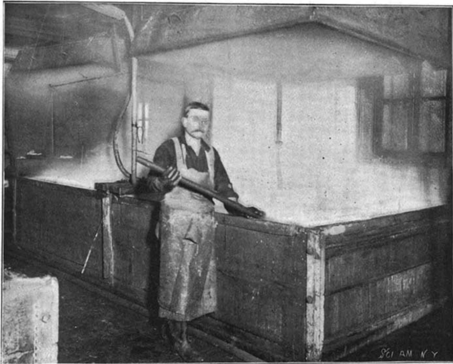
Concentrating the Silver Solution and Precipitating the Silver.
