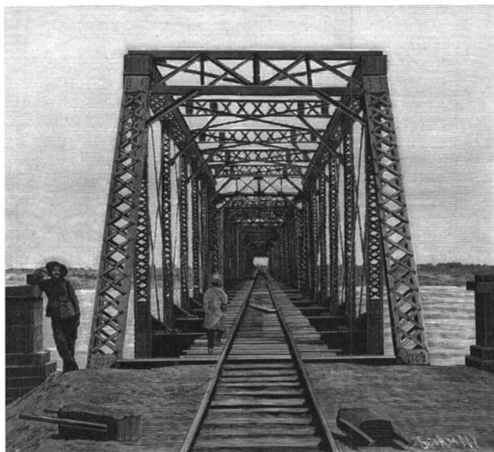
PORTAL VIEW OF THE COMPLETED BRIDGE.
