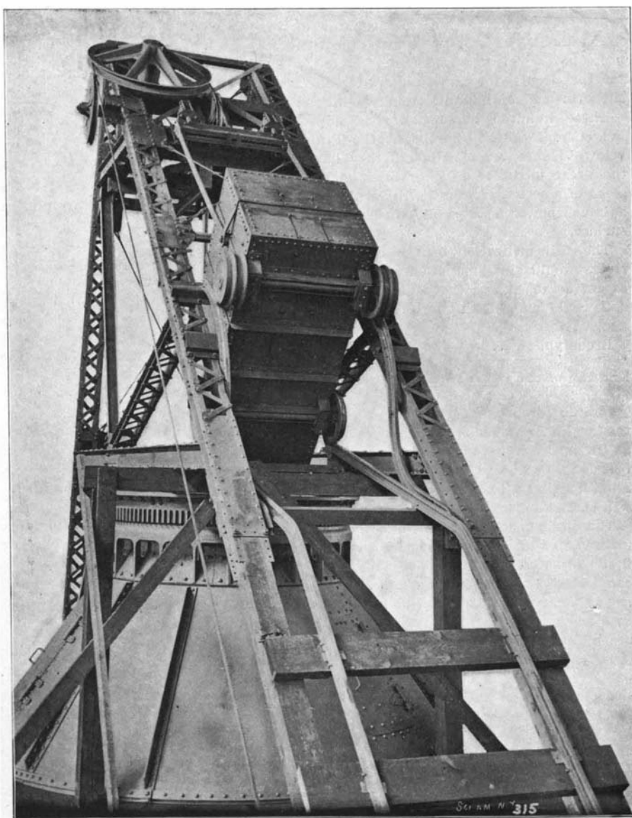
FURNACE HOIST FOR AUTOMATIC CHARGING OF BLAST FURNACES.
