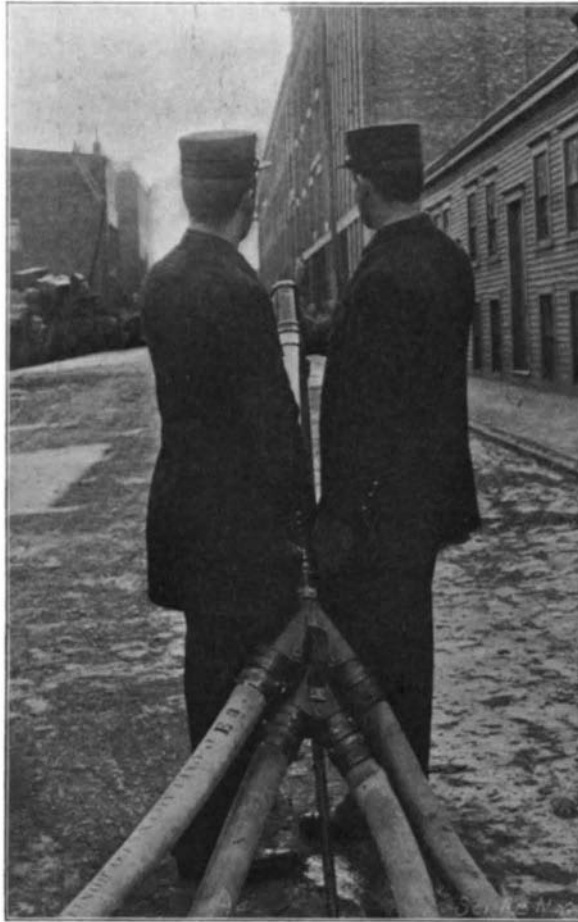
FOUR-WAY CONNECTION ATTACHED TO NOZZLE.
