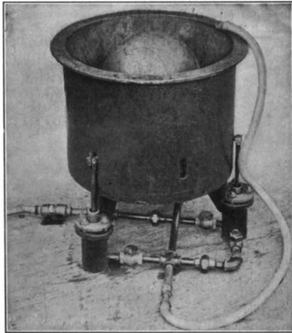
WAVE MOTOR WITH COVER REMOVED.
