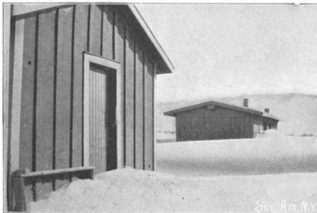
SAND DRIFTS AT RIMLON, CAL.
