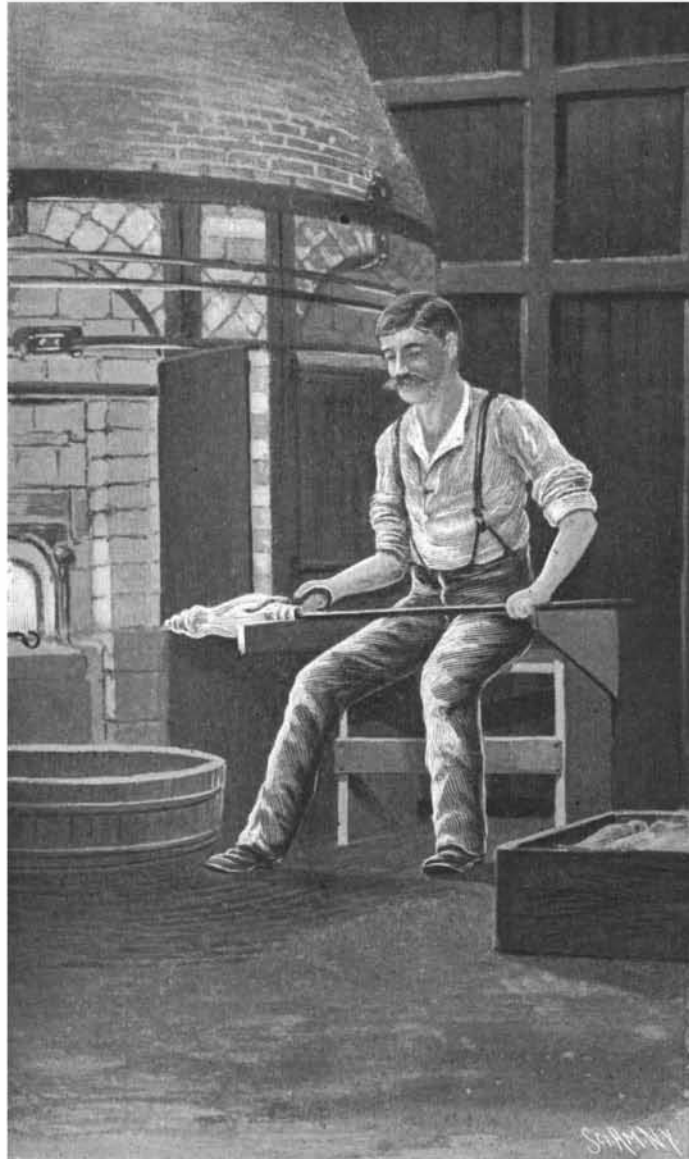
Forming the Ends of the Chimney.
