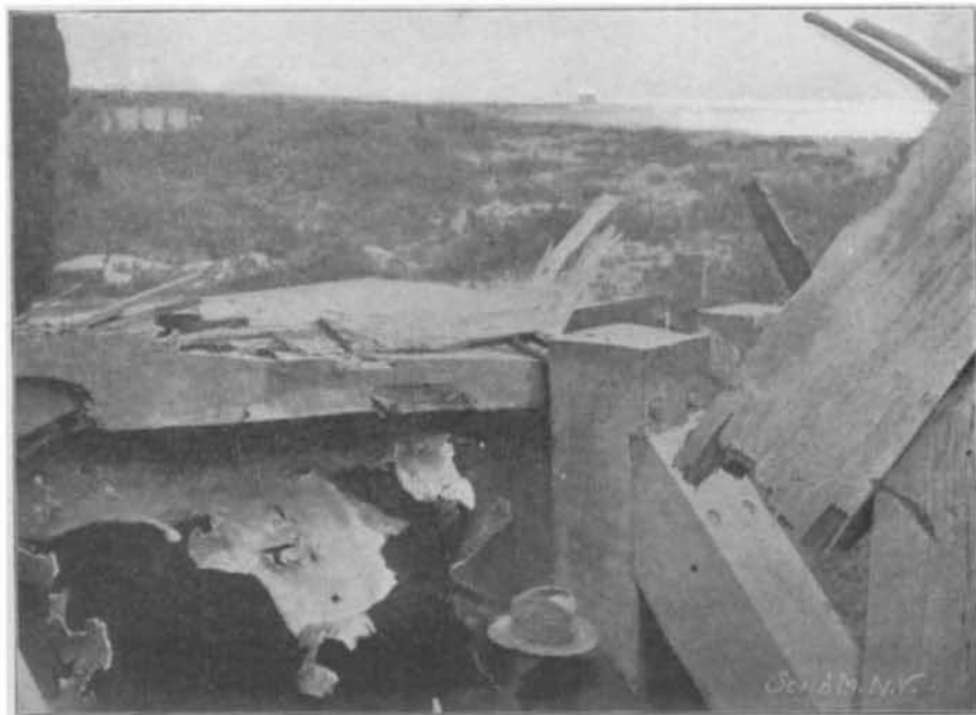
Rear View of Same Target, Showing Complete Destruction Wrought by 12-Inch Armor-Piercing Shot Loaded with 20 Pounds of the New Government High-Explosive.
