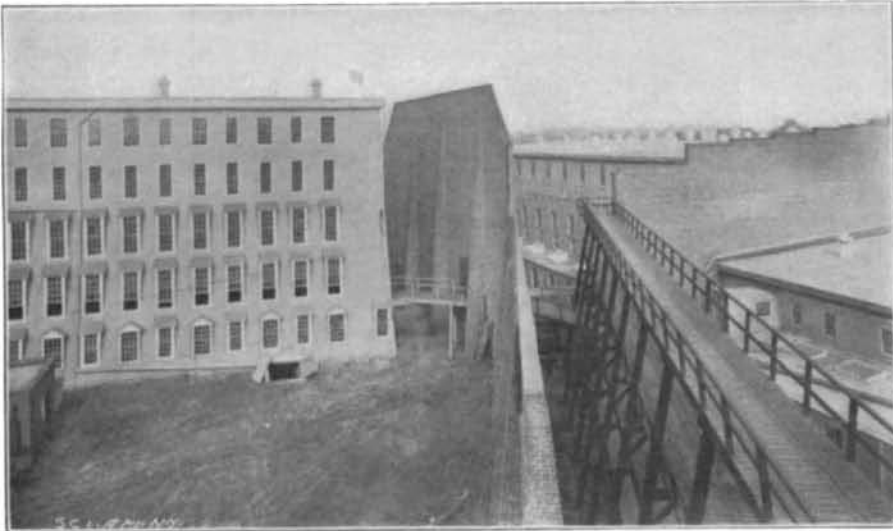
Fire Wall and Railroads.
