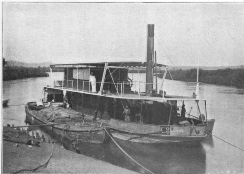
SHALLOW-DRAUGHT STEAMER FOR CONVEYANCE OF MATERIAL FOR CAPE TO CAIRO TELEGRAPH.
