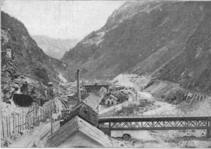
Upper Power House. Iron Bridge Across the Diveria for the Flume. To the Left, a Small Tunnel Leading to the Main Tunnel.
