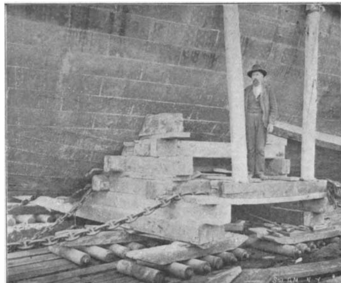
THE ROLLER WAYS ON WHICH THE LIGHTSHIP WAS MOVED.
