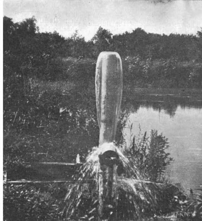
ARTESIAN WELL AT BEAVER CROSSING, NEB.—NINE SUCH WELLS MAKE IT POSSIBLE TO IRRIGATE 115 ACRES.
