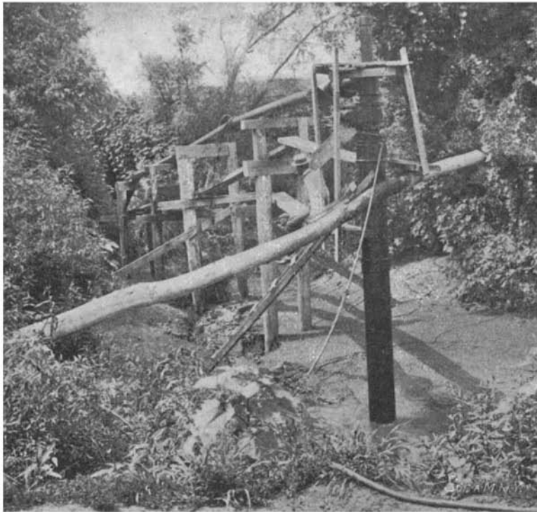
ARTESIAN WELL THAT DISCHARGES 11,158 GALLONS DAILY. DEPTH OF WELL, 1,303 FEET.
