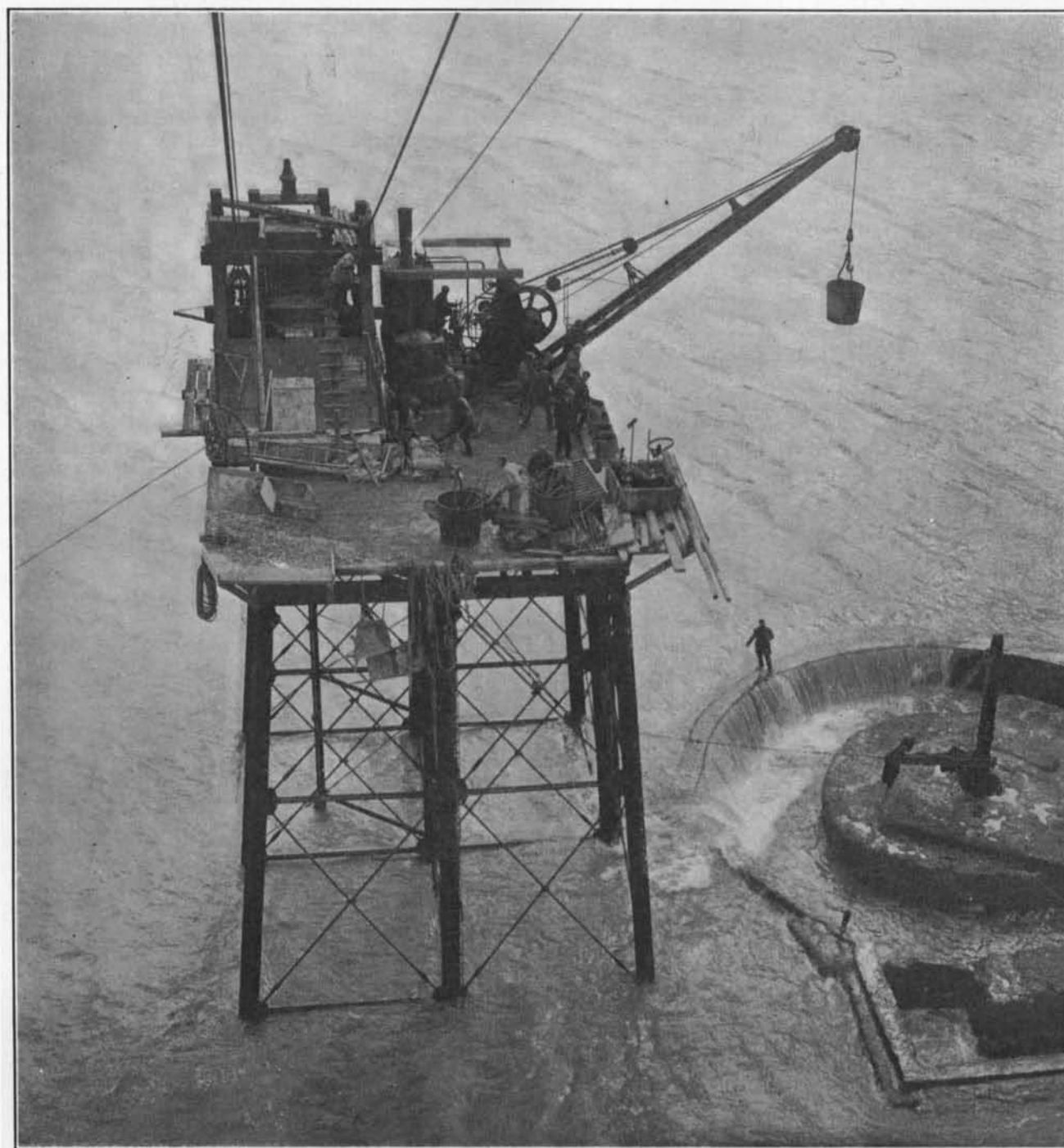
The Erecting Stage and Foundations.
