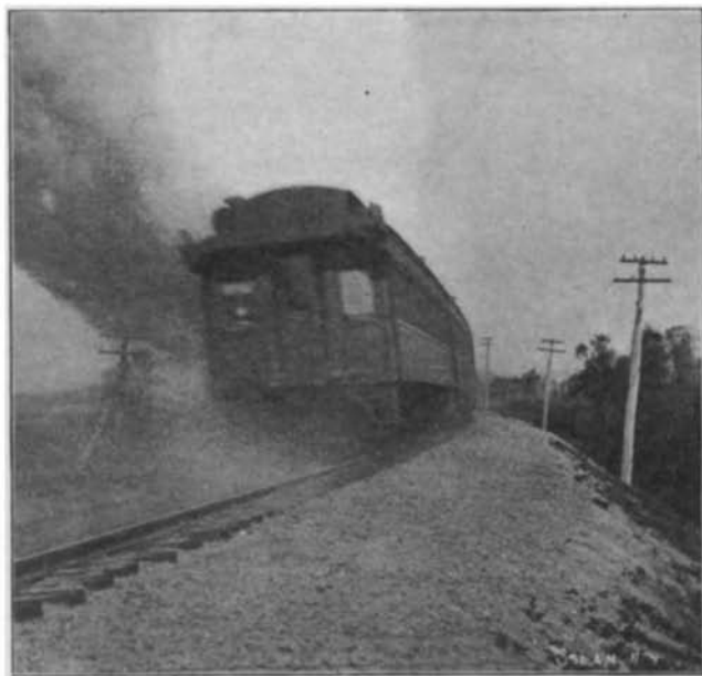
BEFORE OILING, SHOWING DUST RAISED BY EXPRESS TRAIN.
