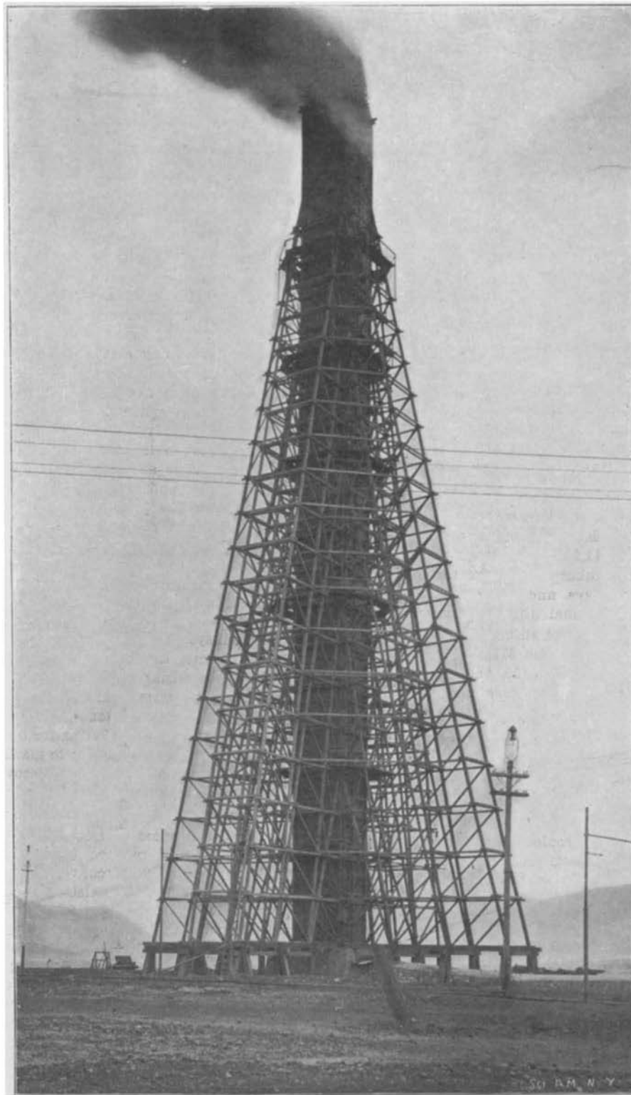
Interior dimensions, 10 feet by 10 feet; height, 180 feet.
