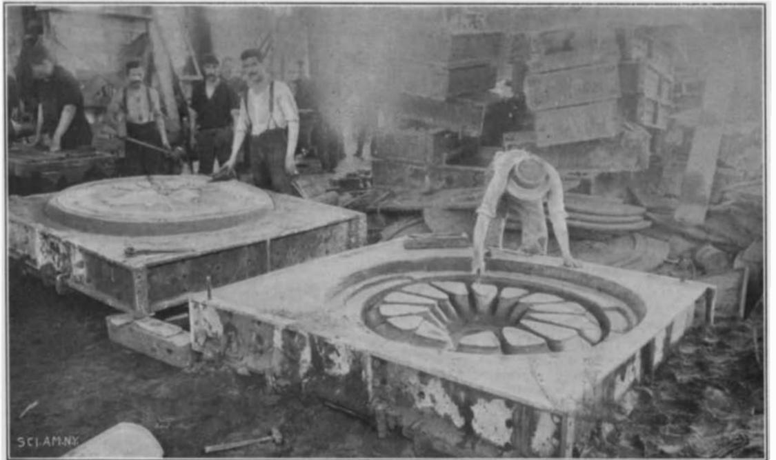
Finishing Mould for Locomotive Driving Wheel.
