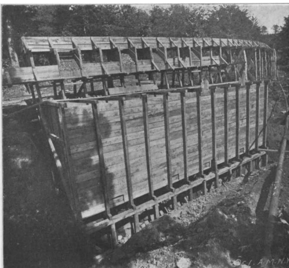
FLUME LINE, GRIZZLIES, ORE BINS, PIPE LINES.
