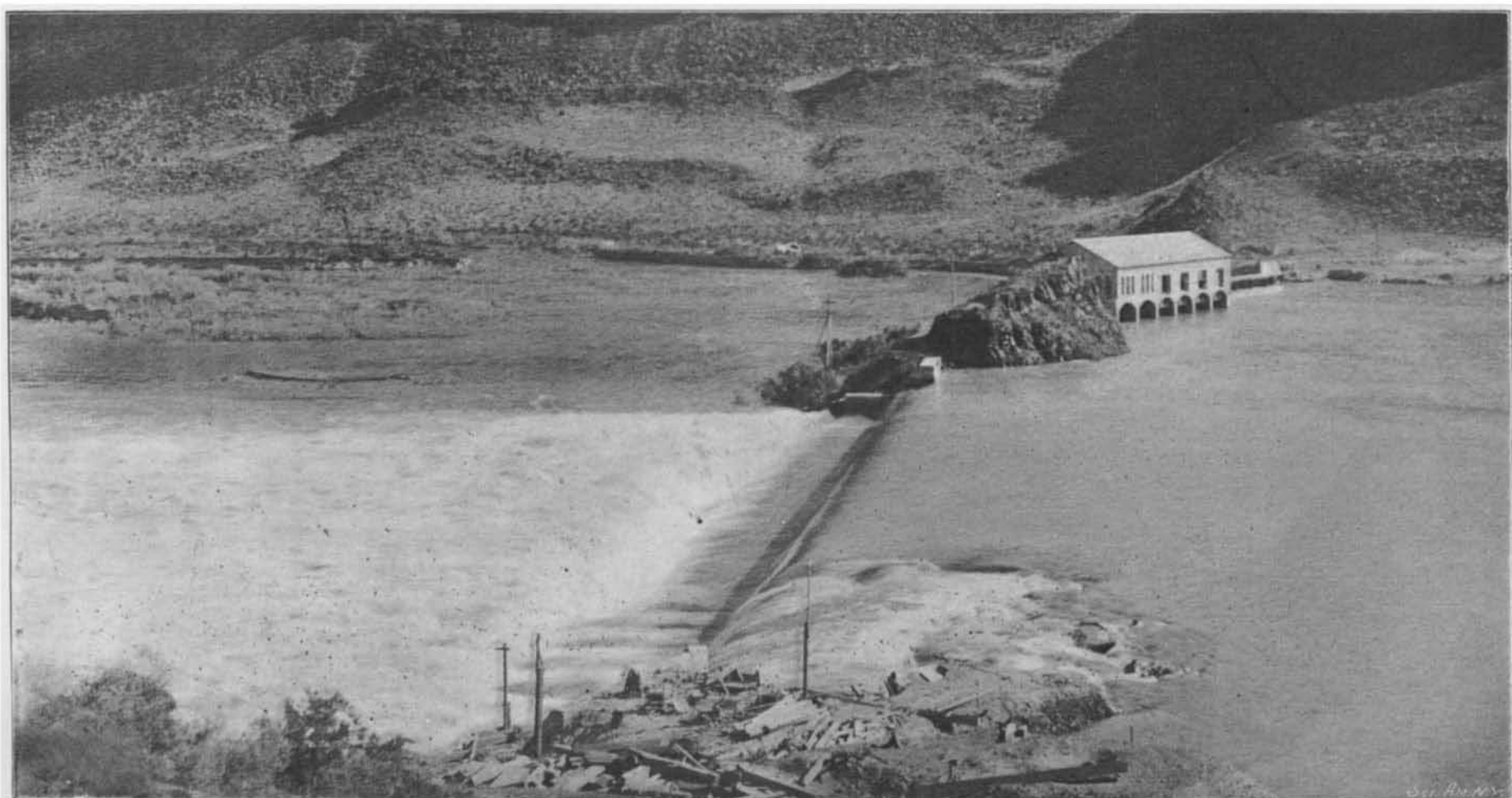
General View of the Dam and Power House.
