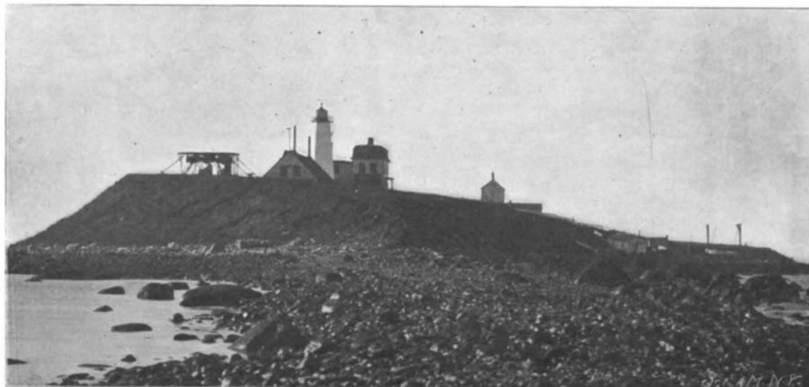
FALKNER ISLAND, LONG ISLAND SOUND, SHOWING FOG-SIGNAL STATION.
