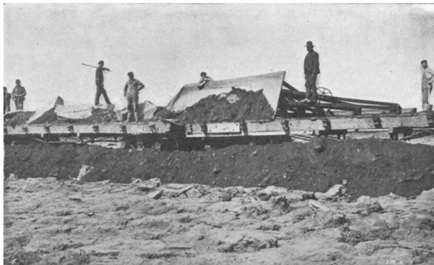
Front View of the Plow, Showing Mold-Board Forcing Load from the Car.
