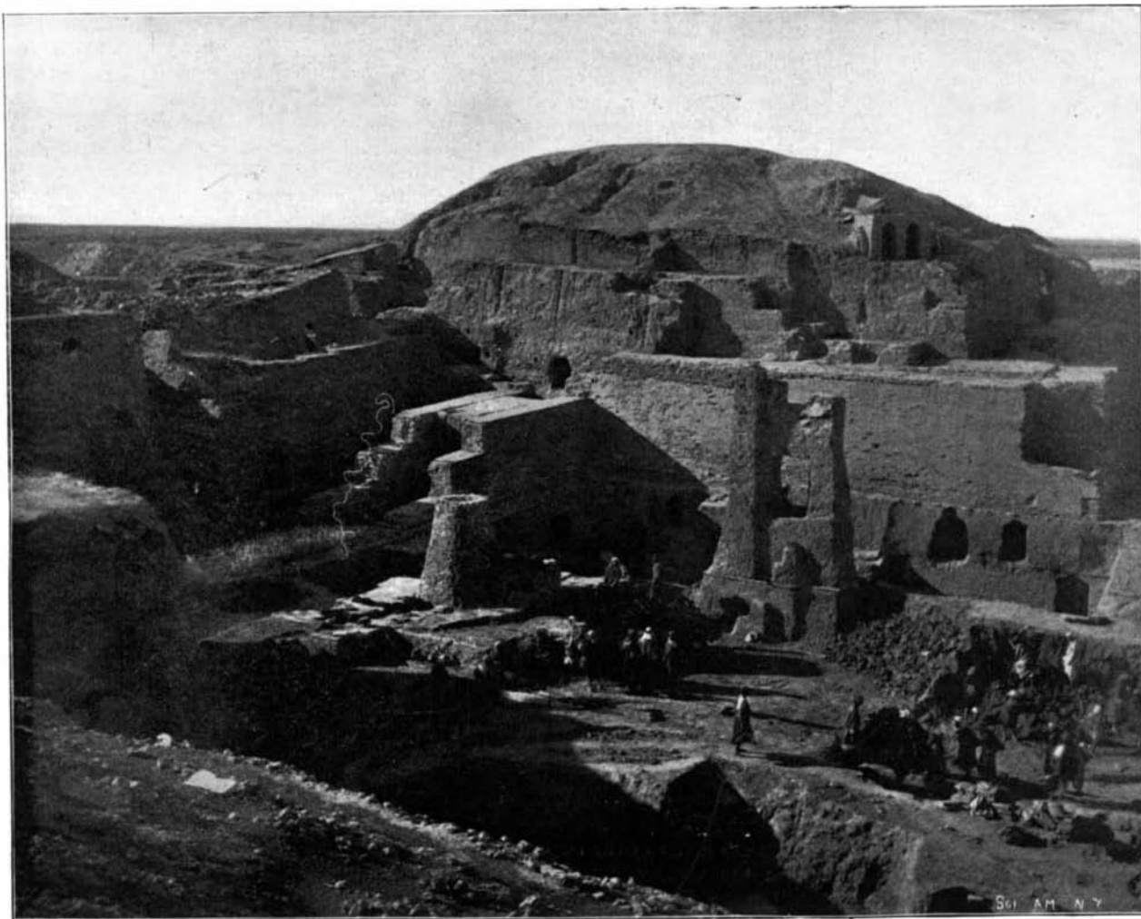
THE STAGE TOWER OF THE TEMPLE OF BEL—WORKMEN ON THE TEMPLE OF SARGON.
