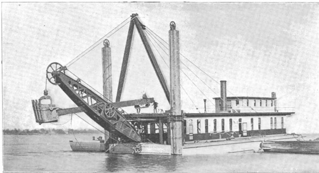
POWERFUL NINE-TON DIPPER DREDGE FOR THE MASSENA CANAL.
