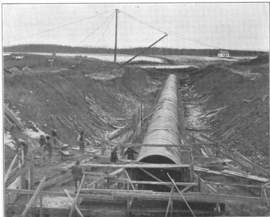
AQUEDUCT FOR CONVEYING GRAISSE RIVER UNDER THE SOULANGES CANAL.
