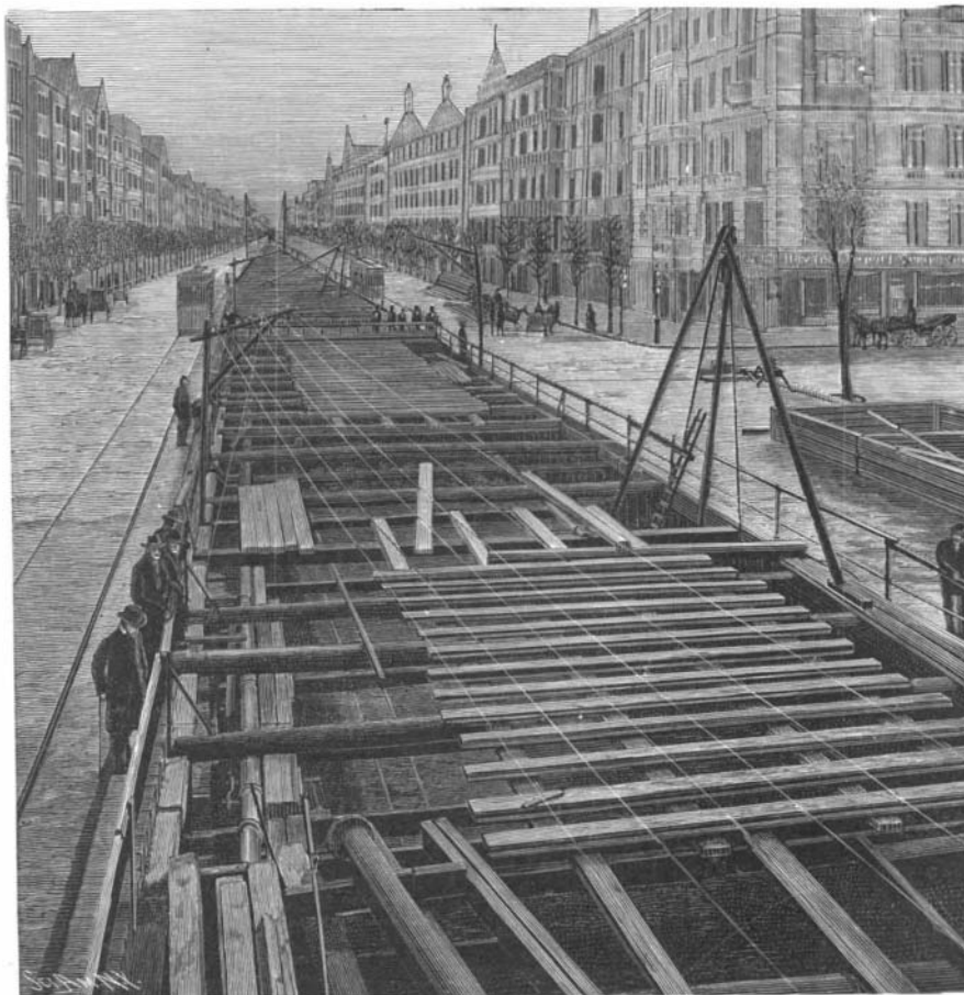
Fig. 2.—EXCAVATIONS FOR BERLIN SUBWAY, SHOWING THE WATER PIPES.
