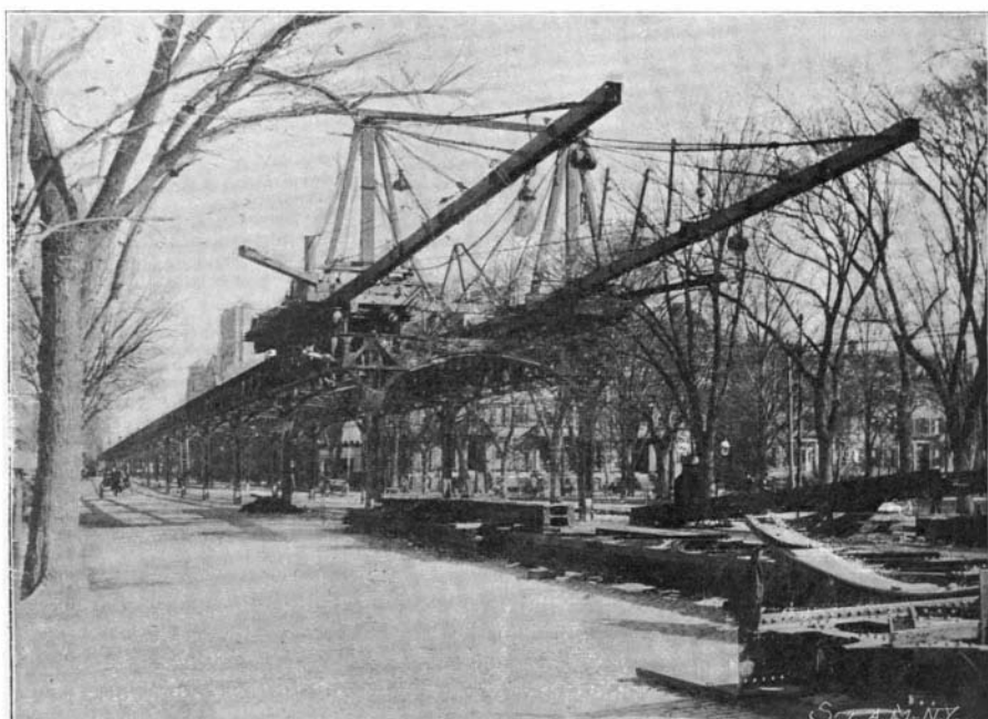
TRAVELER USED IN ERECTION.
