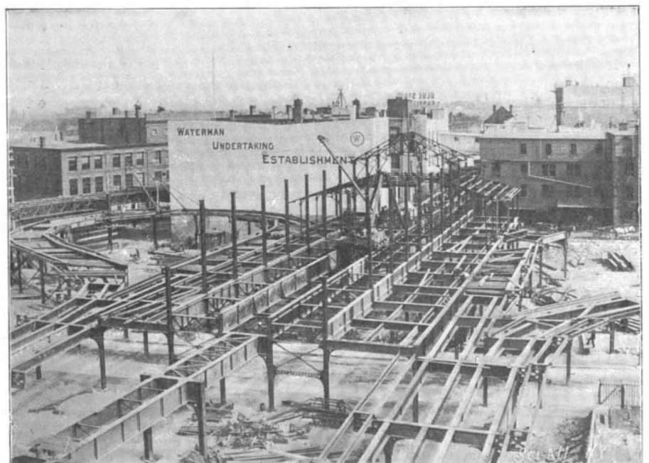
CONSTRUCTION OF DUDLEY STREET TERMINAL.
