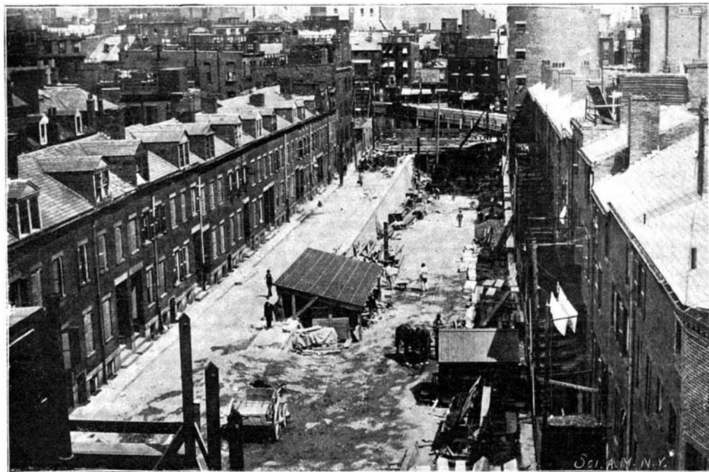
ELEVATED COMPANY'S INCLINE, LOOKING NORTH TO SUBWAY ENTRANCE UNDER PLEASANT STREET.
