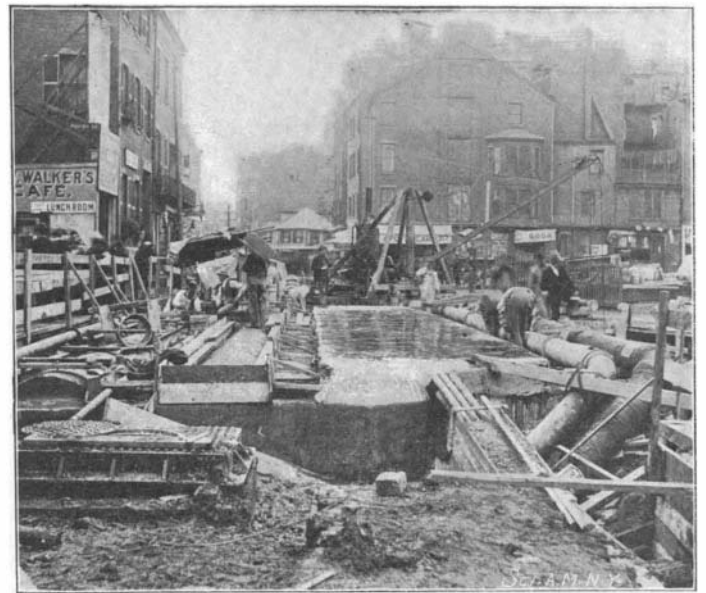
RELAYING PIPES ON SURFACE STREET OVER THE ELEVATED.
