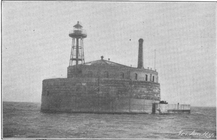
THE INTAKE CRIB COMPLETED.
