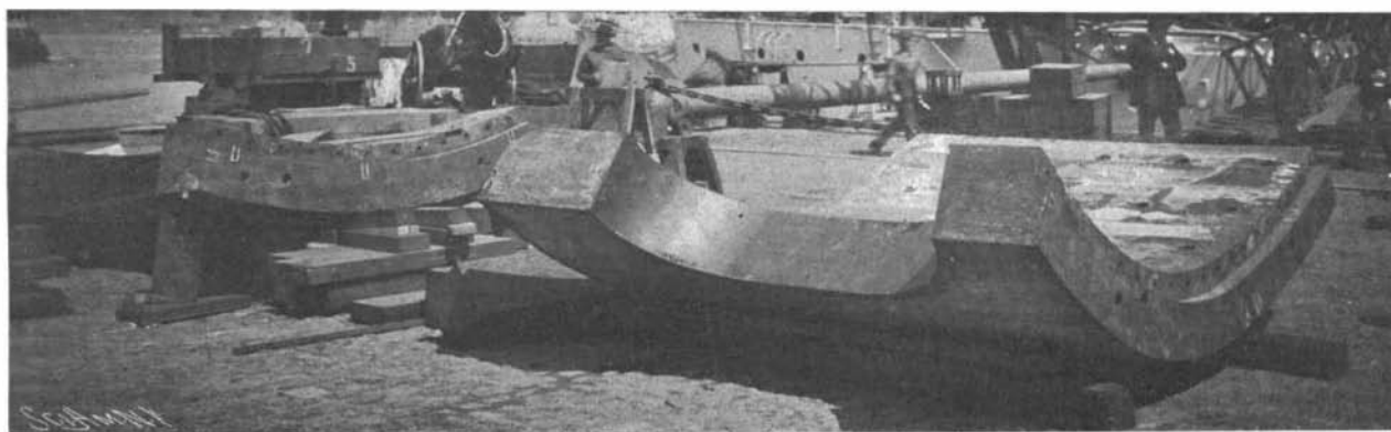
THE 15-INCH AND 17-INCH PORT-PLATES AFTER REMOVAL FROM THE TURRET.
