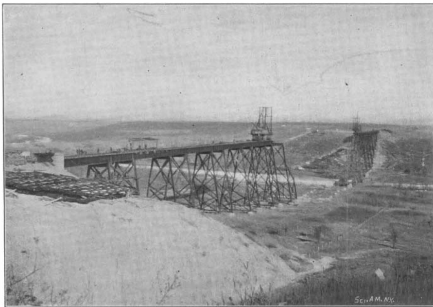
General View of the Viaduct.
