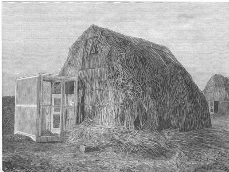
HUT WITH MOSQUITO CAGE AROUND DOOR, WHICH IS ITSELF MOSQUITO PROOF (AS SUGGESTED BY CELLI).
