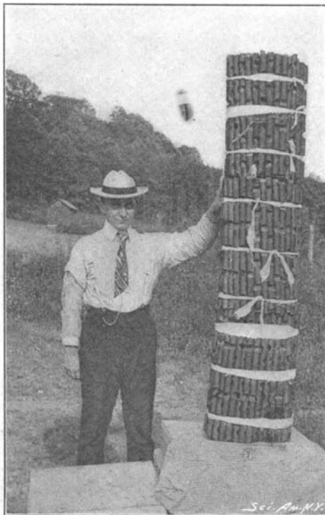
POWDER CHARGE FOR 12-INCH TORPEDO GUN.
