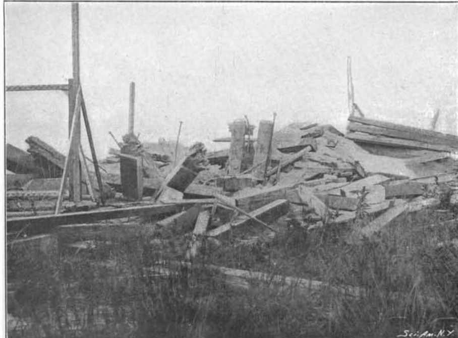
THE TARGET AFTER BEING STRUCK BY GATHMANN 12-INCH SHELL, CONTAINING 200 POUNDS OF WET GUNCOTTON.
