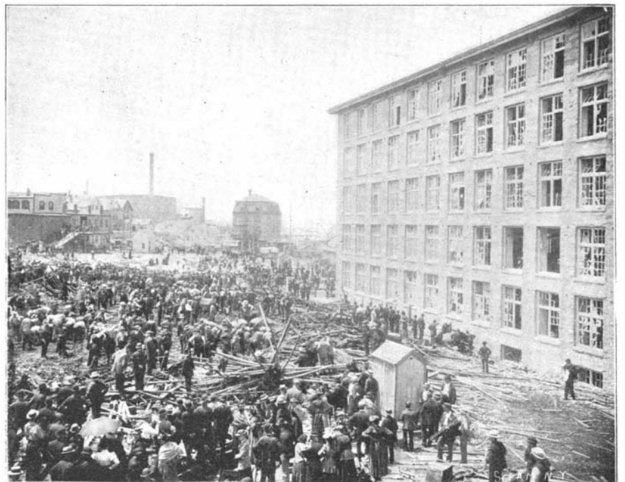
COMPLETE DEMOLITION OF A HARNESS FACTORY BY BOILER EXPLOSION—NOTE BROKEN WINDOWS IN ADJOINING BUILDING.
