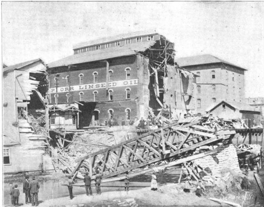
BOILER EXPLOSION AT THE WORKS OF THE NATIONAL OIL COMPANY, PIQUA, OHIO.
