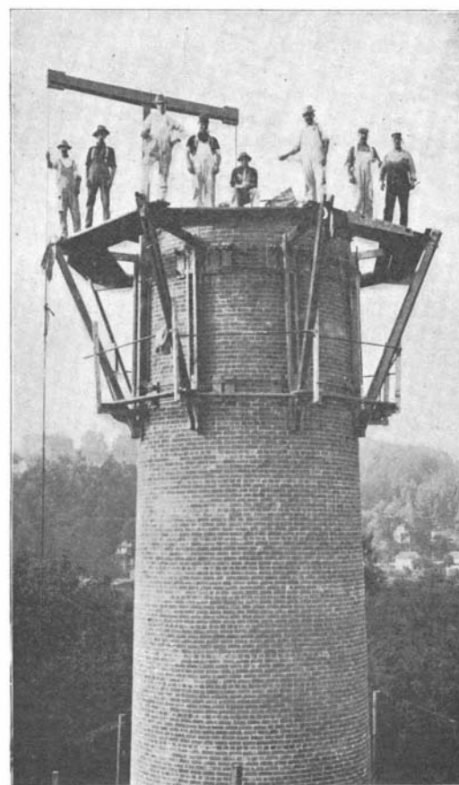
A NEW STAGING FOR BUILDING CHIMNEYS.
