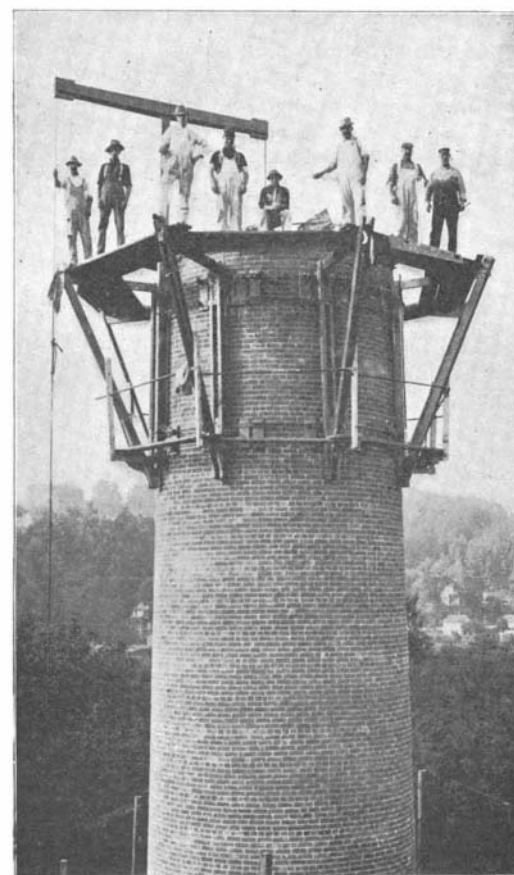
A NEW STAGING FOR BUILDING CHIMNEYS.
