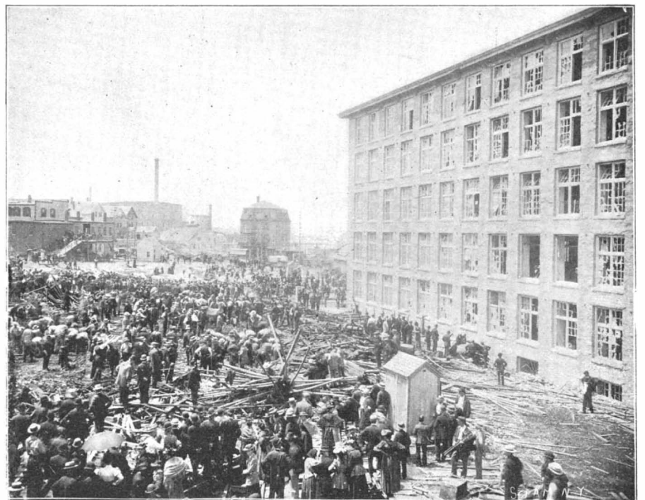
COMPLETE DEMOLITION OF A HARNESS FACTORY BY BOILER EXPLOSION—NOTE BROKEN WINDOWS IN ADJOINING BUILDING.
