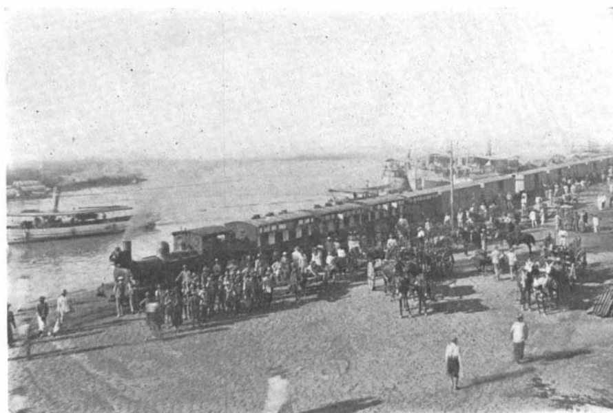
Terminus of the Manila and Dagupan Railway at Manila.
