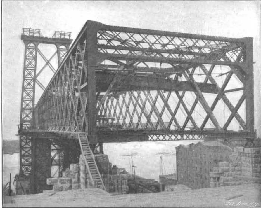
Shore Span from the Brooklyn Anchorage.
