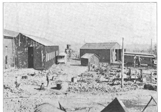
DAMAGE DONE BY BOILER EXPLOSION, SHOWING LOCATION MOTIVE WHICH WAS COMPLETELY STRIPPED.
